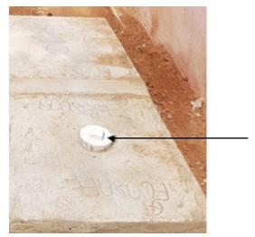
*Plate 57: Cleanout on the cover slap for easy access*
