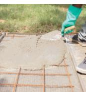
**Plate 20:** Pouring of concrete onto mesh and steel bar setup
