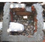
**Plate 54:** Traditional up-flow sand filter
