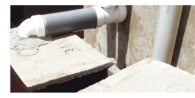
**Plate 46:** P-trap seat connection to Biodigester
