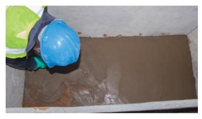
**Plate 29:** Screeding the base of the digester
