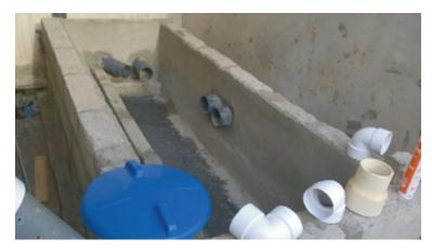
**Plate 38:** Final level of blockwork for Biodigester
