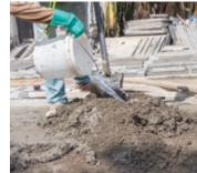
*Plate 15:* Adding on water for concrete
