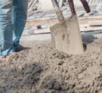
*Plate 16:* Mixing concrete into right consistency 4. Pour concrete into the formwork to occupy half the thickness (depth) of the formwork.
