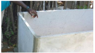
**Plate 28:** Securing biodigester corners with mortar
