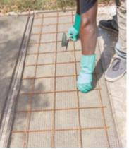
Plate 19: placement of mesh and steel bar setup onto concrete
