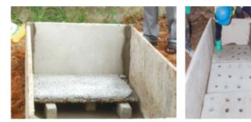
Plate 33: Placement of filter slabs- left: pervious concrete, right: slab with roles
