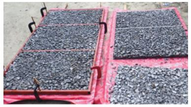
**Plate 24:** Casting of porous slabs
