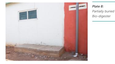
Surface – this installation style is typical in areas with very high-water table and poorly drained soils. In such instances, borrowed soil material, which is well drained, are placed under the Bio-digester. In addition, sand filters are connected to the Bio-digesters for further polishing of the effluent prior to discharge into surface drains and/or water bodies.
