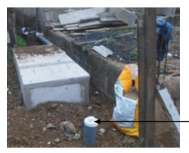
**Plate 58:** cleanout for inspection of buried drain field
