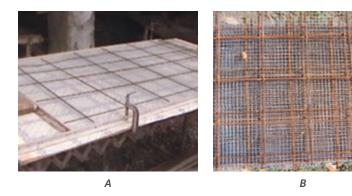
**Plate 13:** Setting out of rebars and chicken mesh
