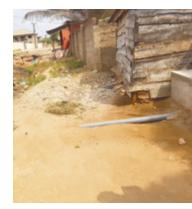
**Plate 42:** Drain field pipe without adequate soil cover
