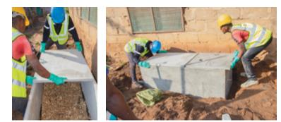
**Plate 36:** Placement of top cover slabs
