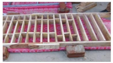
**Plate 22:** Formwork for beam supports for biodigest
