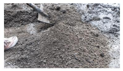
**Plate 14:** Concrete mixture for slabs 2. Mix into a uniform mixture and create a gully in the pile to add on water to the right texture of concrete using a water ratio of 2.0. (Plate 15)
