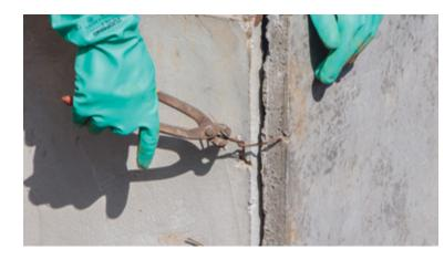
**Plate 27:** How to tie the corners of the Biodigester
