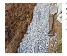
**Plate 53:** covering the perforated pipe with chippings
