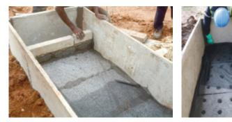
Plate 34: Covering of filter slabs with net.
