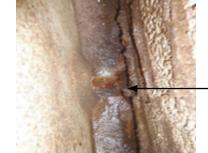
Visible outlet pipe in air gap of Bio-digester (For detection of ponding or blockage)
