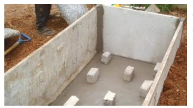
*Plate 32: Placing of concrete beam supports.*   Place the two (2) porous slabs/perforated concrete slabs on the concrete beam to create an air gap between the screeding and the porous slab; there is always about 6 inches space between the laid porous slabs and the bio-digester box.
