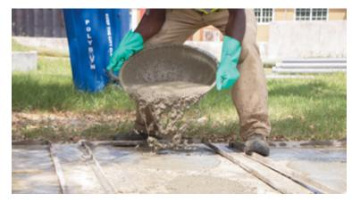
**Plate 17:** Pouring of concrete into formwork
