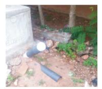
**Plate 41:** Short drain field pipe less than designed length
