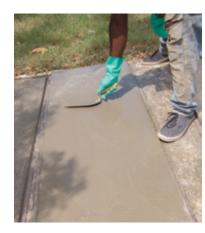
**Plate 21:** Working concrete to a smooth surface finish
