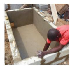
**Plate 39:** Rendering of inside wall of Bio-digester
