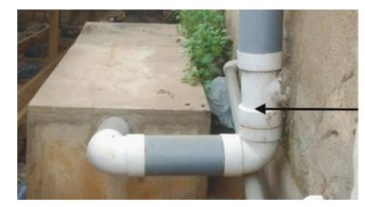
Plate 49: influent pipe from toilet seat and vent pipe
