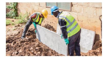
**Plate 26:** Forming the Biodigester box from the slabs.
