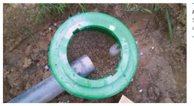
**Plate 6:** Sand filter installed in a poorly drained area
