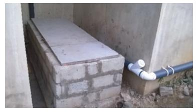
Plate 40: Blockwork biodigester before outside rendering
