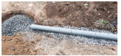
**Plate 52:** Laying of perforated pipe on bed of chippings
