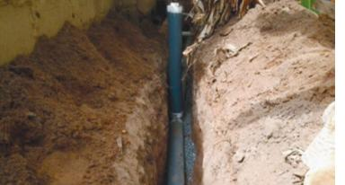
**Plate 31:** Pipe drain field installation
