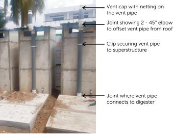
Plate 50: Vent pipe through the exterior wall
