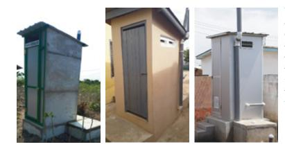
Plate 44: left: Concrete superstructure, middle: blockwork superstructure and far right: alucobond superstructure.
