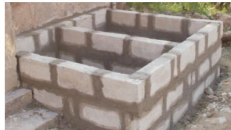
**Plate 37:** Blockwork for Bio-digester
