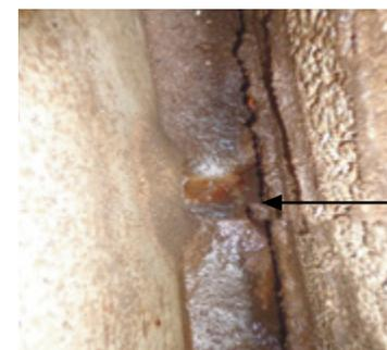
Visible outlet pipe in air gap of Bio-digester (For detection of ponding or blockage)
