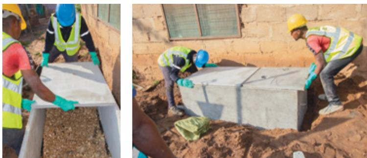
**Plate 36:** Placement of top cover slabs
