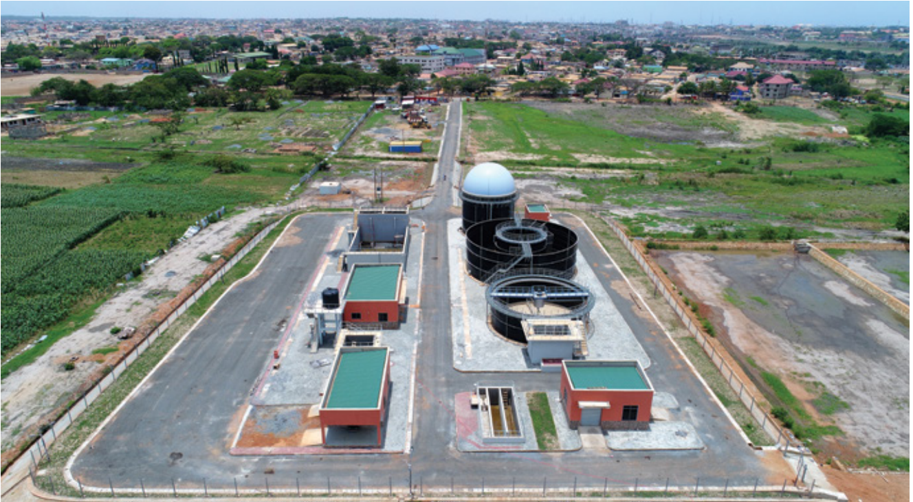
Simplified Sewerage System at Ashaiman New Town in the Ashaiman Municipality
