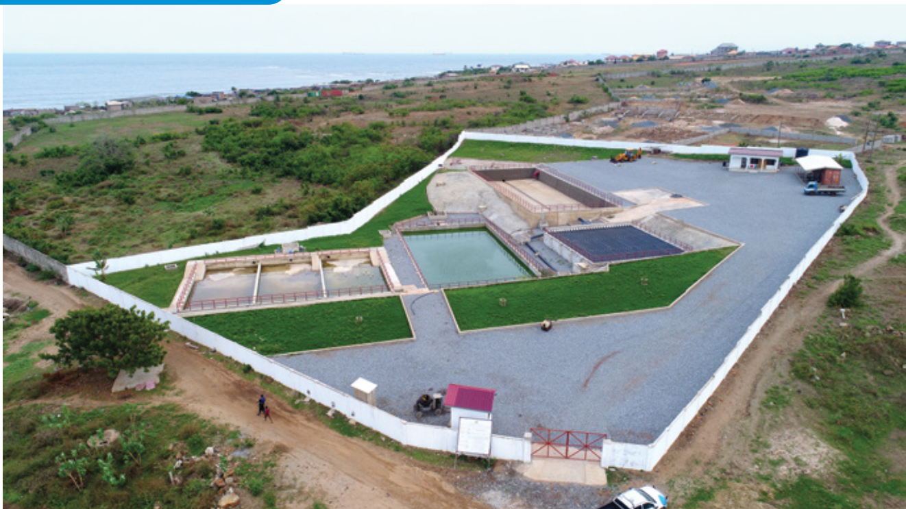
Simplified Sewerage Treatment Plant at Bankuman in the Tema Metropolis
