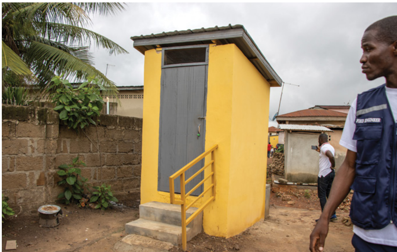
A completed stand-alone household toilet at Ejisu Besease.
