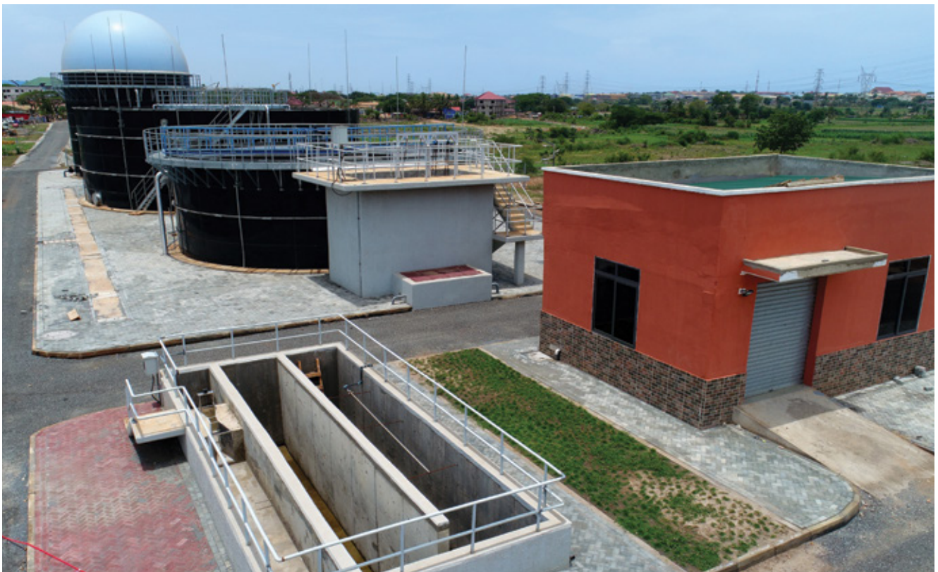
A view of some components of the Ashaiman Facility
