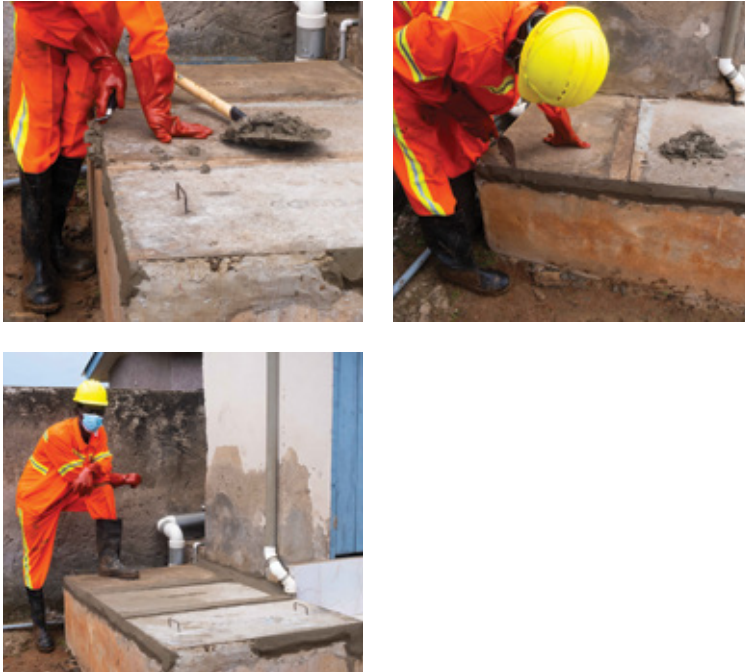
Figure 16: Sealing the cover slab with mortar after opening for emptying
