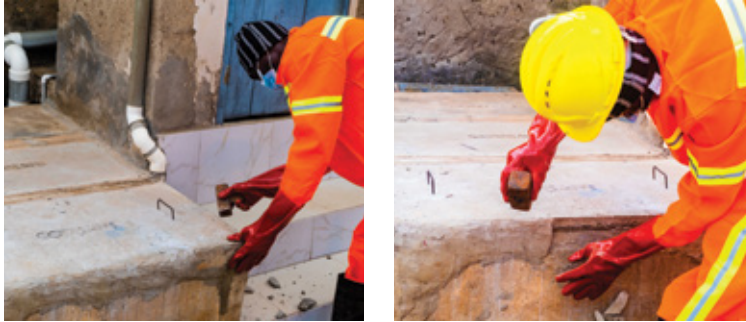
Figure 4: Biodigester emptier carefully chiselling off mortar to open the biodigester
