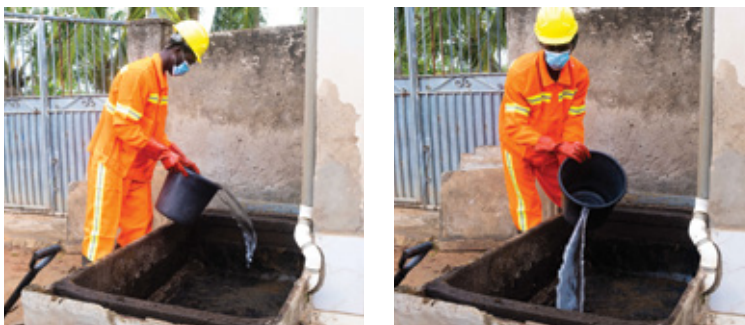
Figure 11: Washing the digester by pouring water directly from the bucket.
