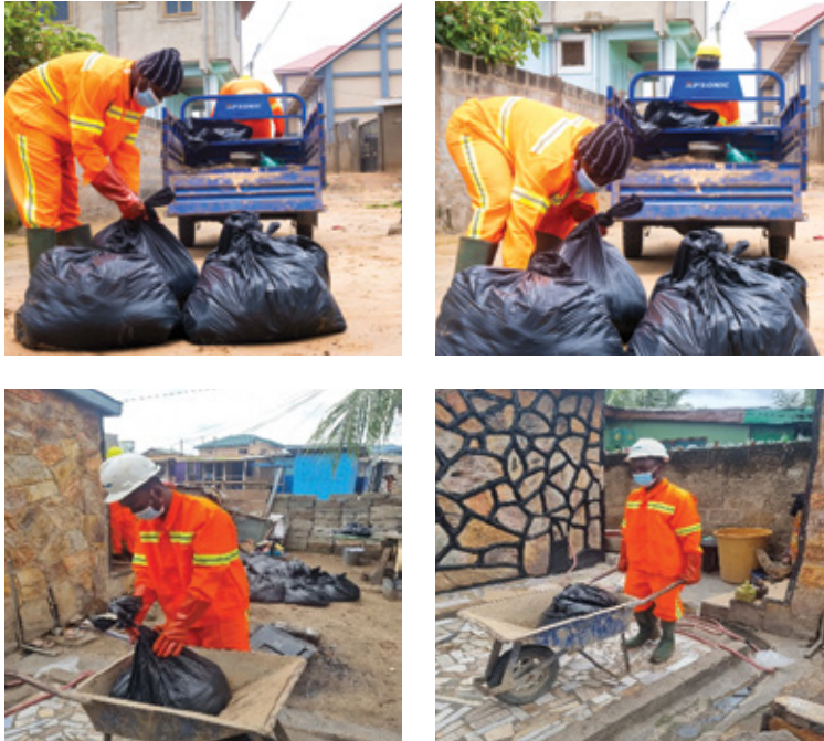
Figure 17: Transporting Scooped sludge off the site.
