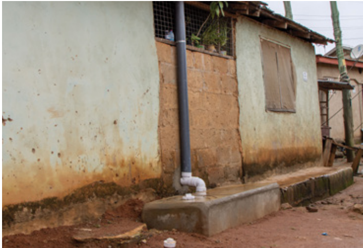
Figure 2: Digester only toilet
