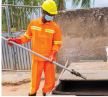
Figure 7: Some sludge stick to the dipstick showing moisture content is okay for emptying
