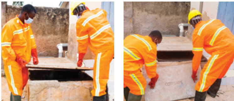
Figure 5: Cover slab of biodigester being taken off.
