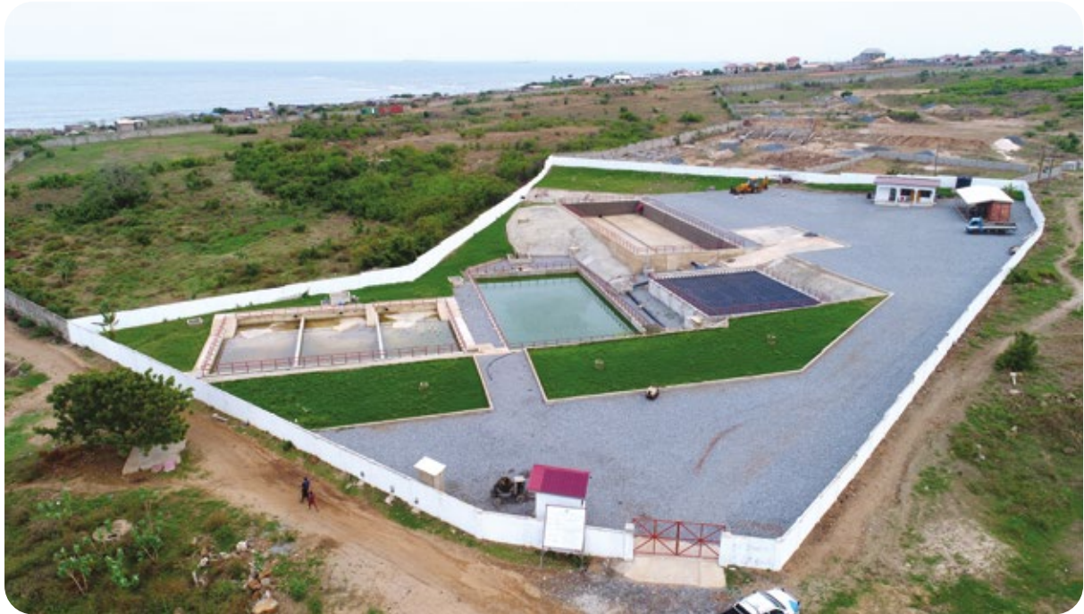
Simplified Sewerage Treatment Plant at Bankuman in the Tema Metropolis
