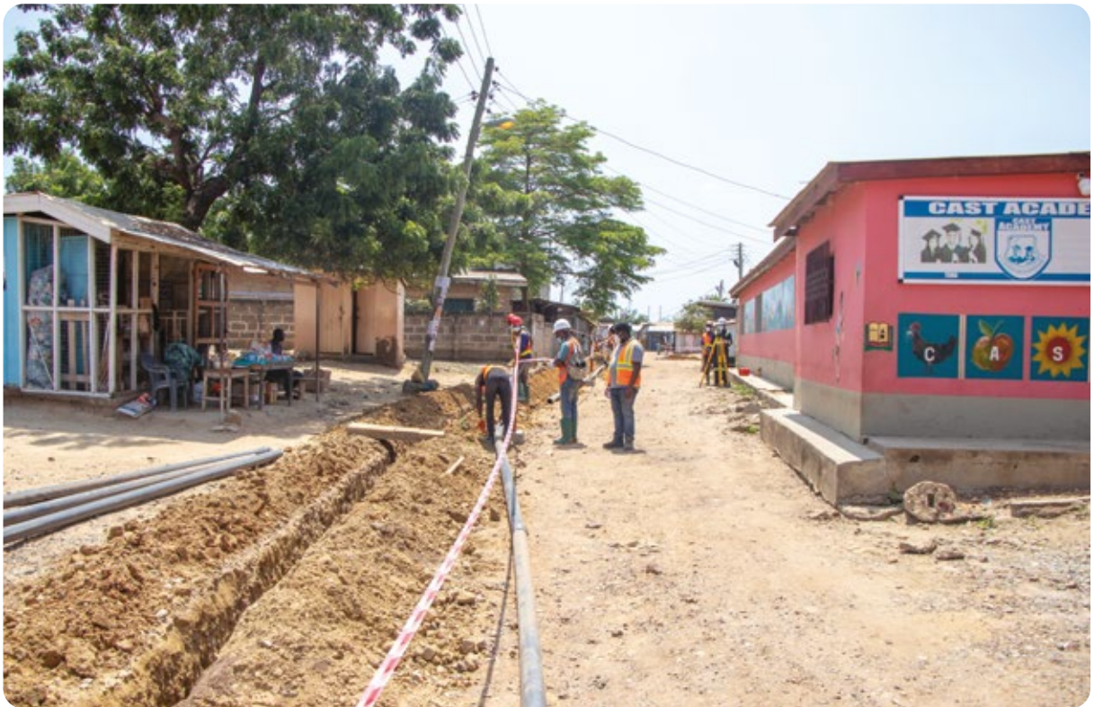
Households in Bankuman being connected to sewer lines
